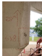
Figure 6: Typical Delaminated Area
