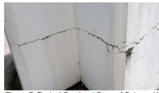
Figure 7: Typical Cracks at Base of Column (4)
